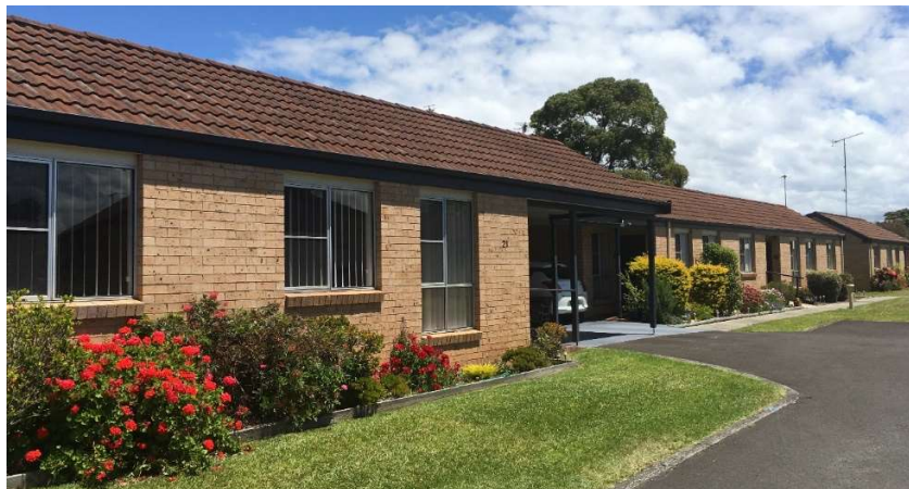
Figure 4-1: Warrigal Warilla Village units current ‘meantime use’ for skilled migrant workers
